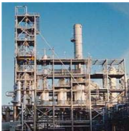
Modern Aromatics Complex with BTX-Sulfolane Unit
